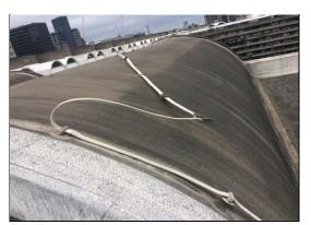
2. In many areas, lightning strips need to be re-fixed. This is evident on many of the Barrel roof areas.
