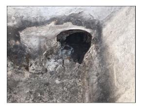
15. <u>Andrewes House Barrel Roof Areas</u> Liquid has de-bonded from the concrete upstand with cracking also evident causing water ingress.
