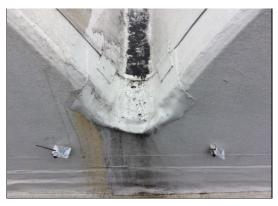
Close up of the existing lead and gutter that has been painted/coated.
